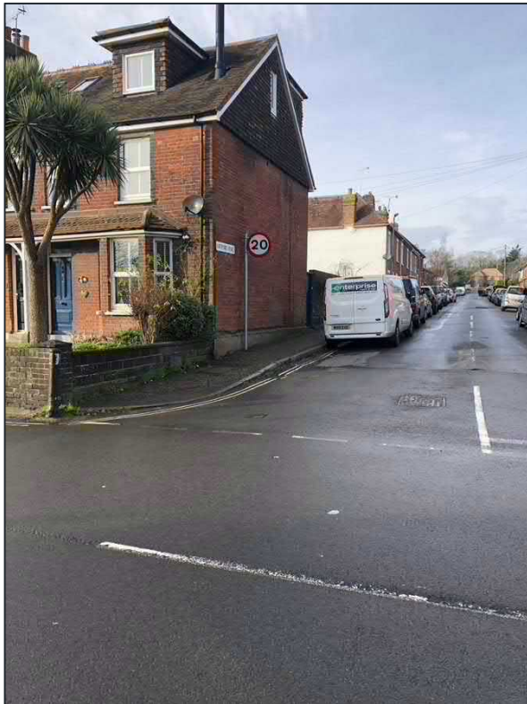
Figure 3-16 - Side road junctions with poor visibility in Section 3
