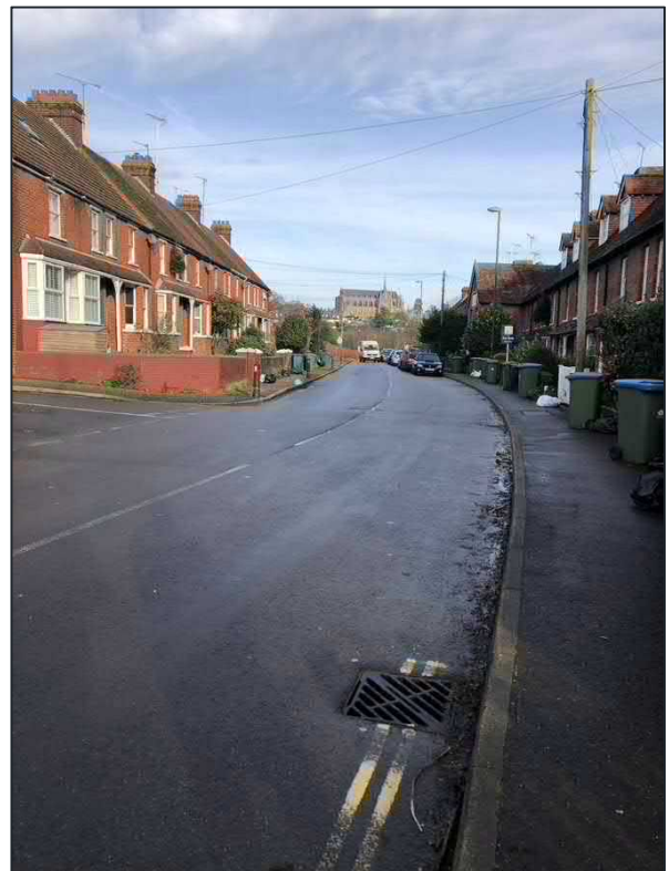
Figure 3-15 –Restricted road width in Sec. 3
